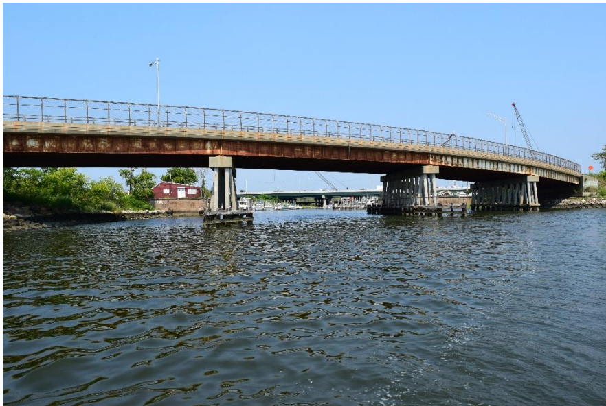
Photo 2-7: Kimberly Ave. Bridge looking upstream on the West River
