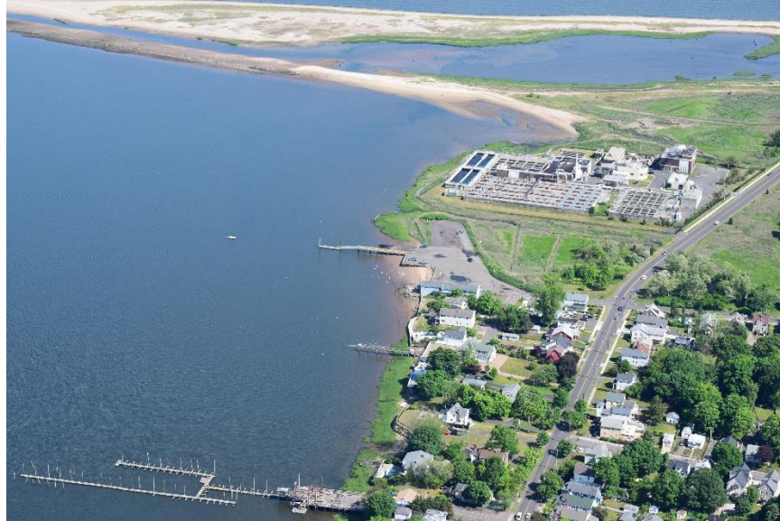
Photo 4-1: Water Pollution Control Plant on 1 st Ave. near Sandy Point, adjoining April St. boat ramp.
