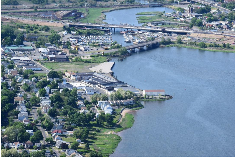
Photo 7-2: West River Crossing and Haven South Redevelopment Area
