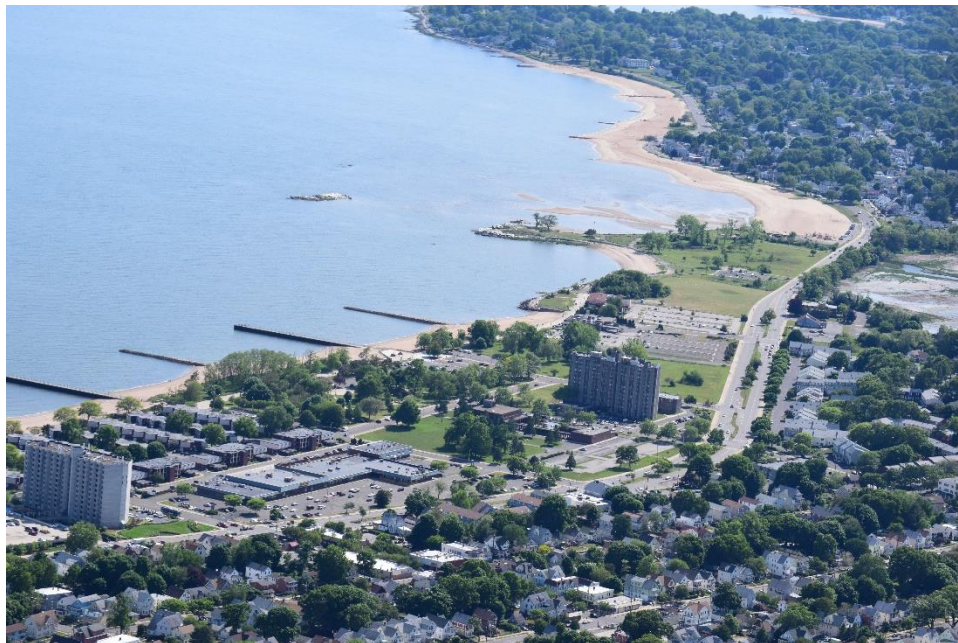
Photo 7-4: West Haven Beaches and Cove River
