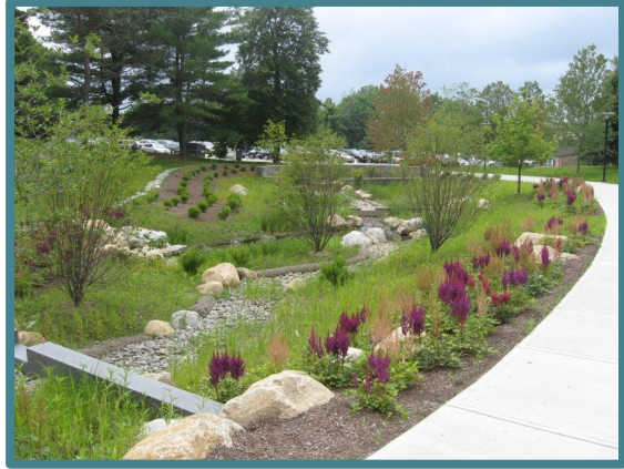
Rain Gardens and Bioretention System
