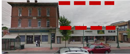
Figure E – Roof Parapet and Cornice Lines
